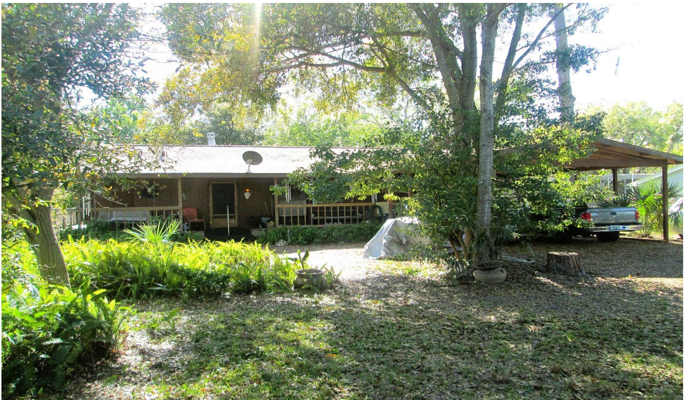
Front yard, facing south towards front of existing residence and carport improvement
