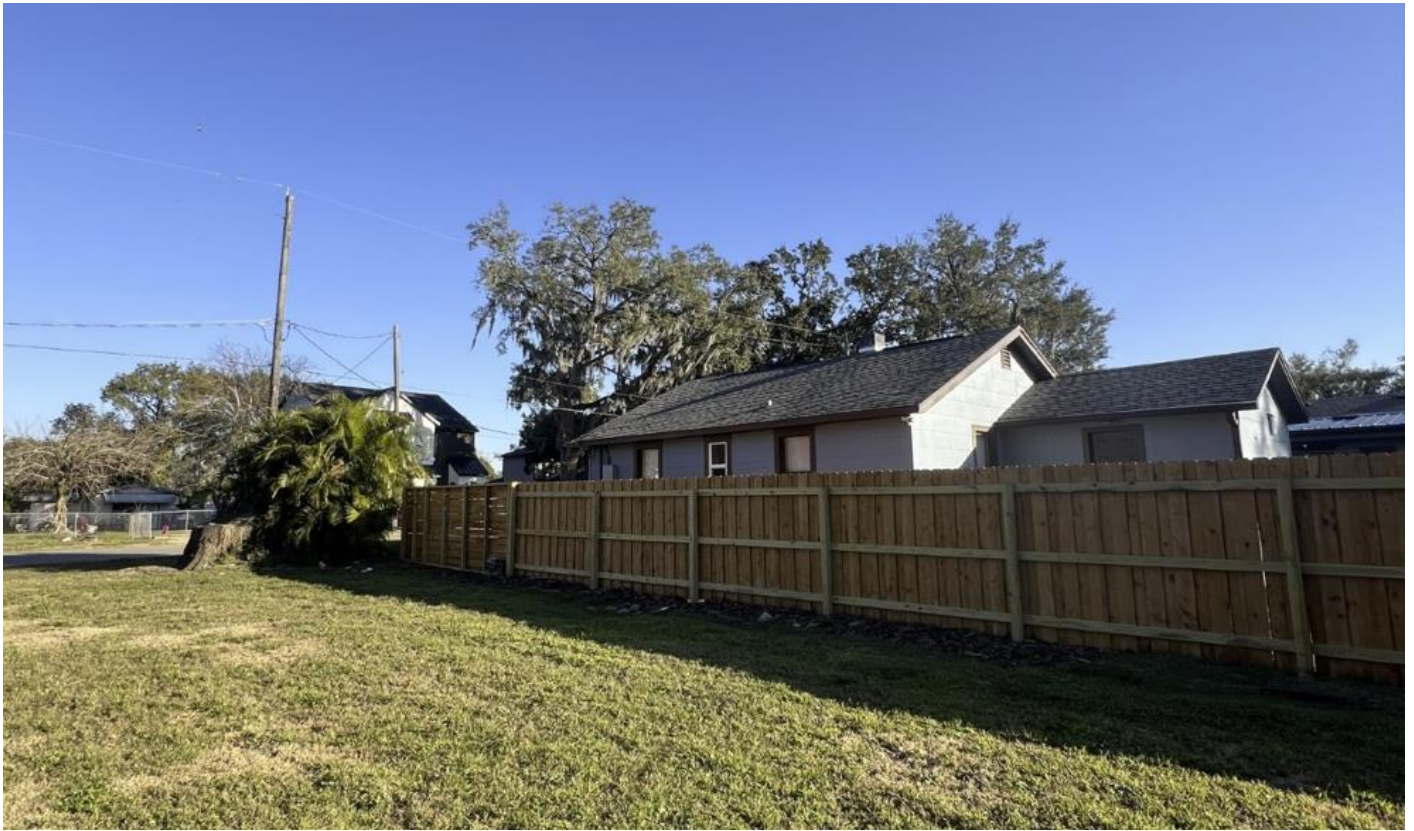
Facing southwest towards the neighboring property to the south
